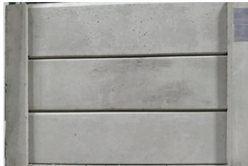
PRECAST SLABS 1 440 x 300mm
